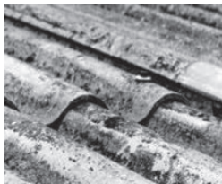
Super Six Asbestos Roof
